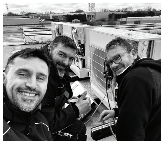
New air conditioning systems
