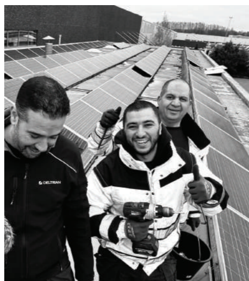
Installation of solar panels
